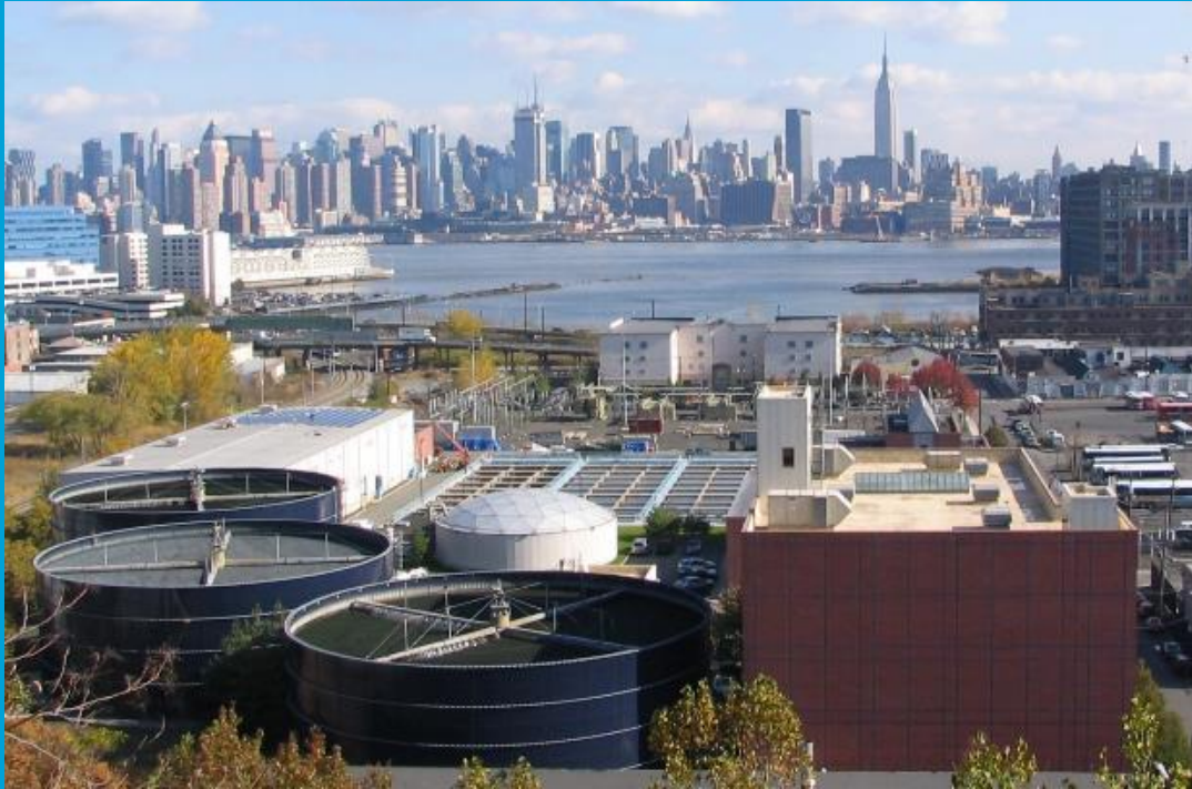
Adams Street Wastewater Treatment Plant 1600 Adams Street, Hoboken 20 million gallons per day (MGD)
