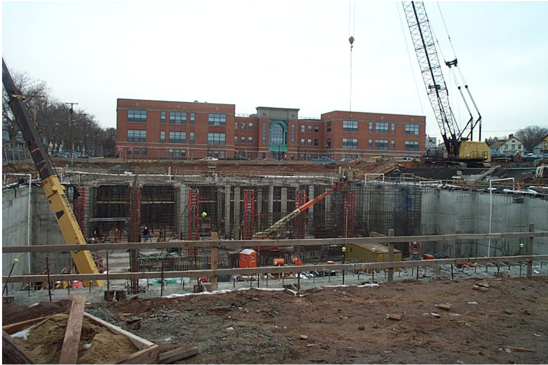
Truman School in New Haven, CT CSO Storage Tank beneath parking lot
